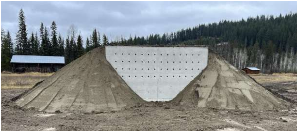
Figure 6. Bank Swallow structure at Spike Elk Farm/Moberly Marsh showing front view with perforated holes in cement slabs and nesting substrate banks on the sides.
