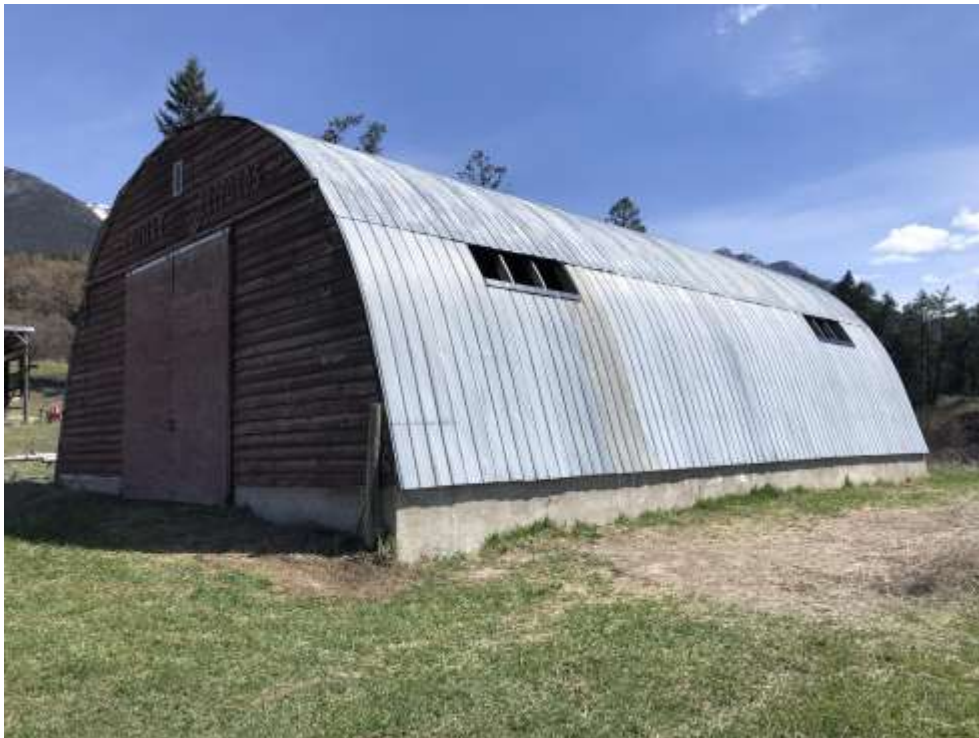
Figure 8. Edgewater Quonset structure repaired and enhanced to increase habitat availability for bats and Barn Swallows.
